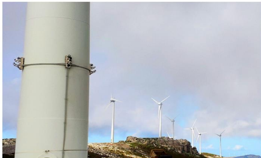
Installation of a Bird Monitoring System at the Jasper Energy Wind Farm in Stavros Evia
